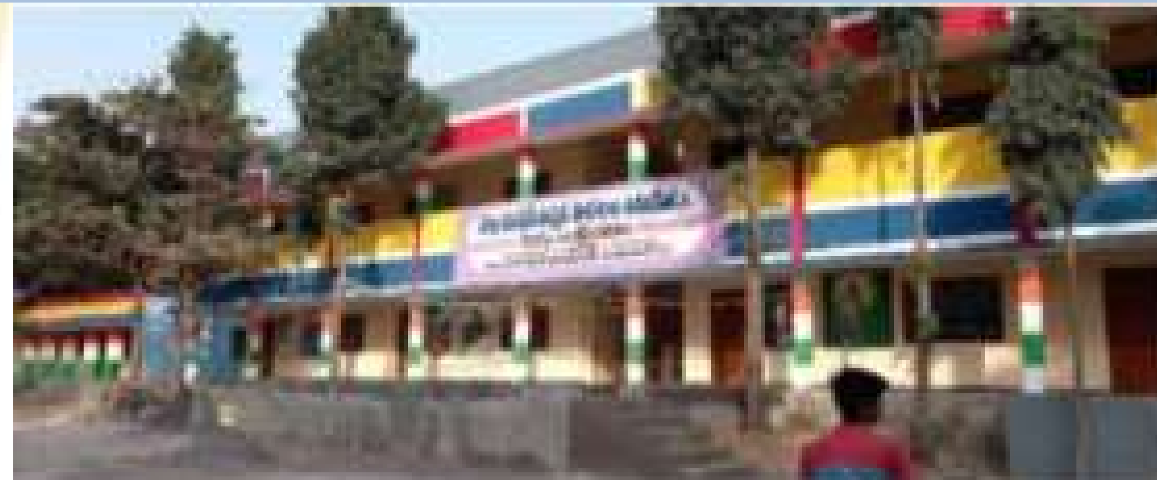
School building after repair work
