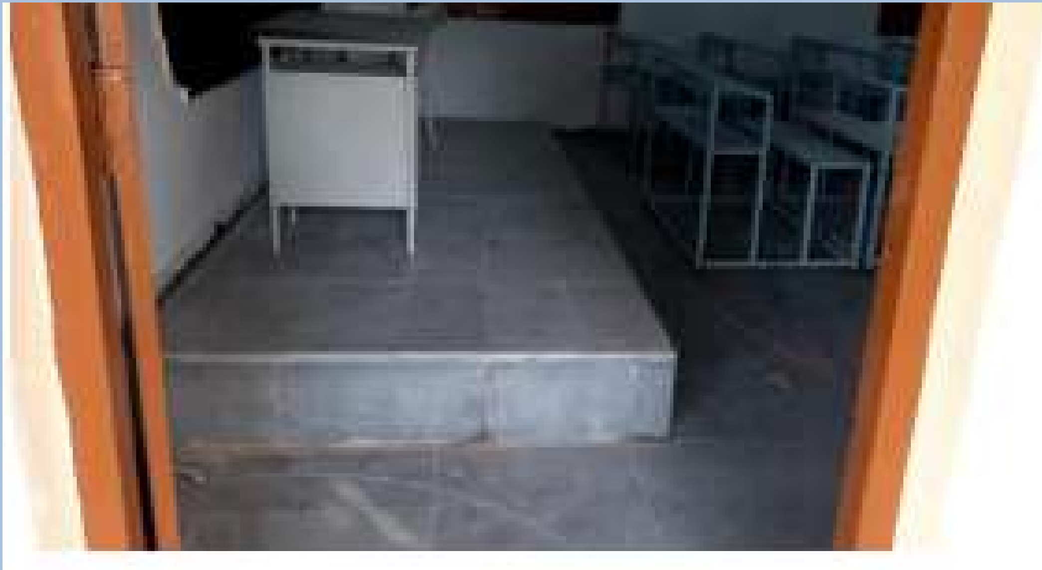
Classroom flooring work with tandoor stones
