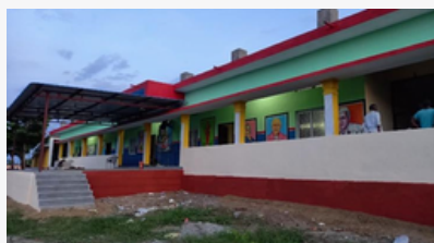
After classroom repair
