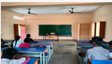
After classroom repair with tandoor tiles
